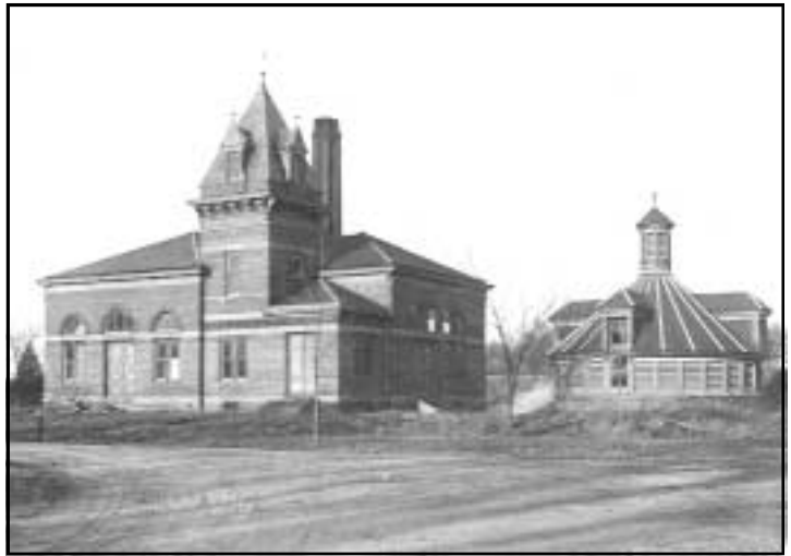
Water Works Pumping Station, December 9, 1898.
