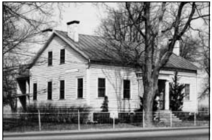
White Star Tavern, home of Adam & Elizabeth Gartner, near the present intersection of Route 159 and Route 23, north of Chillicothe, near the current hospital. This home was built c. 1800, and was once used as a stagecoach stop. It was later owned by the Fischer & Vaughn Families, descendants of the Gartner's. It was razed in 1956, for the widening of U.S. Route 23.
